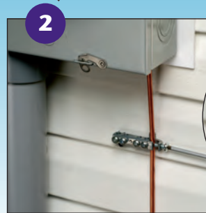
2 Insert grounding electrode conductor into the lay in lug. Tighten screw.
